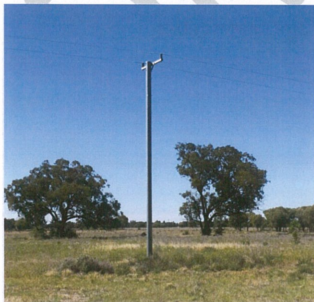
Photograph 3: Overhead powerline situated on the subject site
